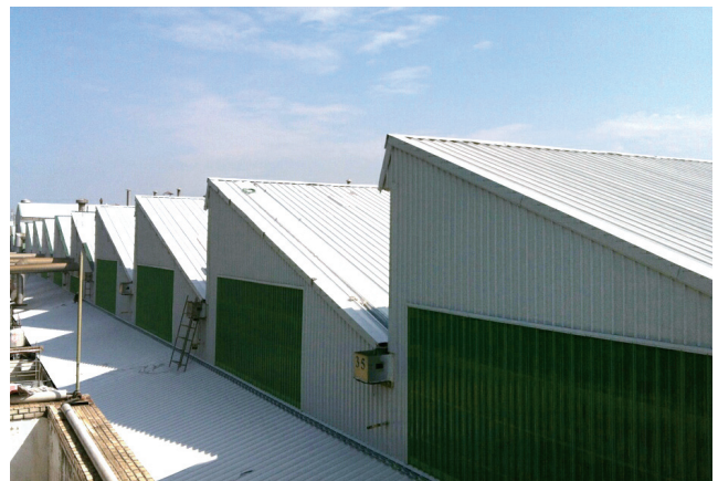
苗栗縣裕隆汽車廠房 鍍層量 Y27，PVDF 塗料 Plant building of Yulon Motors, Miaoli, Taiwan Coating mass: Y27; paint type: PVDF
