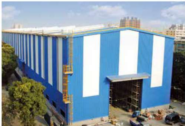
高雄市中鋼機械廠房 鍍層量 Y30，PE 塗料 Plant building of China Steel Machinery Corp., Kaohsiung, Taiwan Coating mass: Y30; paint type: PE
