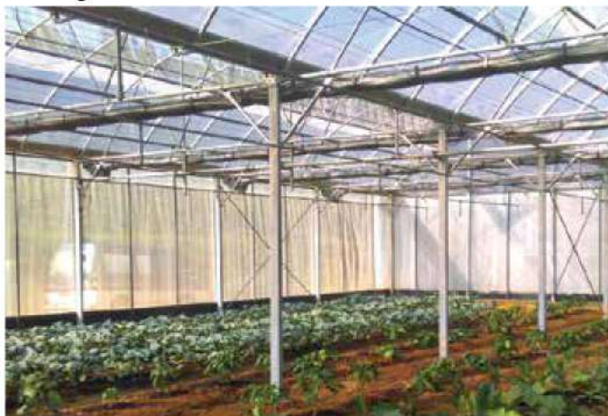
溫室支架管，鍍層量 Y35 Steel tube supporters for greenhouse Coating mass: Y35
