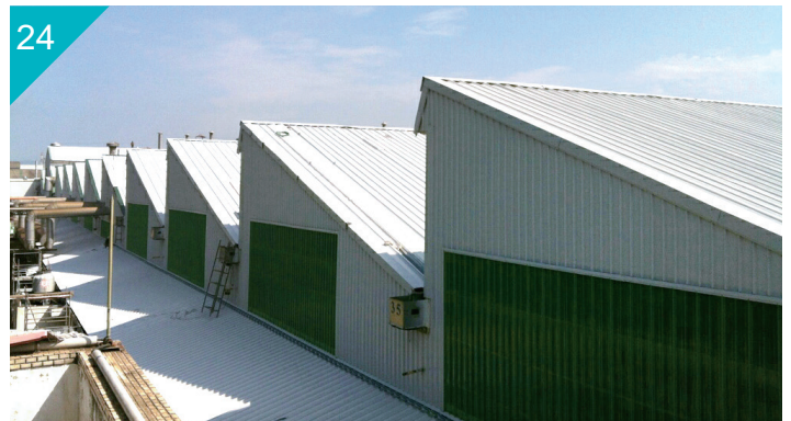
苗栗縣裕隆汽車廠，PVDF 烤漆鋼板 Plant Building of Yulon Motors, Miaoli, Taiwan Paint Type: PVDF
