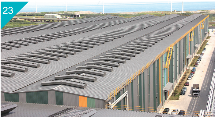
桃園縣東和鋼鐵企業(股)公司屋頂 / 外牆，PVDF 烤漆鋼板 Roofing/Siding of Tung Ho Steel Enterprise Corp., Taoyuan, Taiwan Paint Type: PVDF
