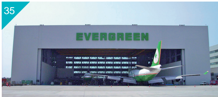
桃園長榮航太(股)公司第三飛機維修棚廠屋頂 / 側牆，PVDF 烤漆鋼板 Roofing/Siding of the 3rd Hangar of Evergreen Aviation Technologies Corp., Taoyuan, Taiwan Paint Type: PVDF
