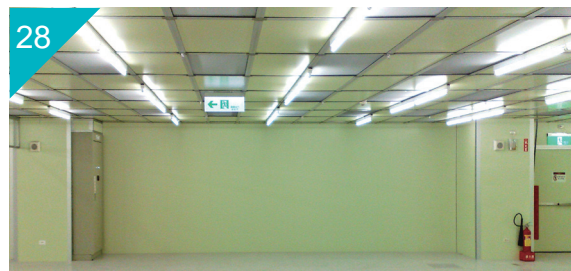
日月光中壢廠房抗靜電無塵室，抗靜電烤漆鋼板 Clean Room of Advanced Semiconductor Engineering Inc., Jungli, Taiwan Anti-Electrostatic Polyester Pre-Painted Steel Sheet
