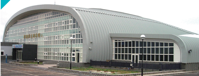
澎湖縣立游泳館屋頂 / 側牆，PVDF 烤漆鋼板 Roofing/Siding of Penghu County Swimming Pool, Penghu, Taiwan Paint Type: PVDF
