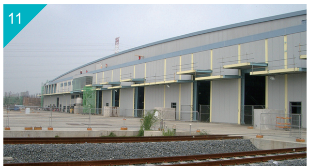
11 台灣高鐵高雄燕巢總機廠屋頂 / 側牆，PVDF 烤漆鋼板 Roofing/Siding of Taiwan High Speed Rail-Yenchao Main Workshop, Kaohsiung, Taiwan Paint Type: PVDF
