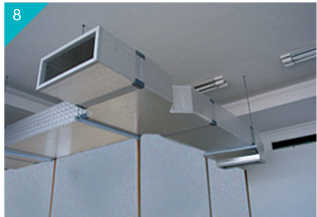
8 空調風管，抗菌鍍鋅鋼板 Ducting Anti-Microbial Metallic Coated Steel Sheet
