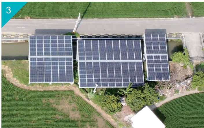
3 彰化田中 (大排, 地面型), 使用熱浸鍍 5% 鋁鎂鋅鋼板 Tianzhong Township, Changhua County (Ditch, Ground type) Hot-Dip 5% Al-Mg-Zn Coated Steel Sheet
