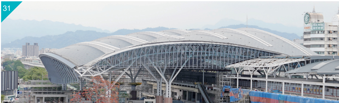
台灣鐵路管理局台中車站屋頂，PVDF 烤漆鋼板 Roofing of Taichung Train Station of Taiwan Railways Administration Paint Type: PVDF
