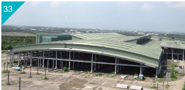
屏東縣潮州台鐵客車及機車維修廠屋頂 / 側牆，PVDF 烤漆鋼板 Roofing/Siding of Taiwan Railways Administration Chaozhou Coach Yard, Pingtung, Taiwan Paint Type: PVDF
