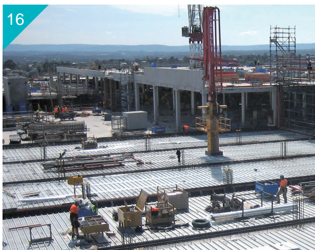
樓承板 (澳洲墨爾本皇家兒童醫院實照) 熱浸鍍 5% 鋁鋅鋼板 Floor Decks of the Royal Children's Hospital in Melbourne, Australia Hot-Dip 5% Al-Zn Coated Steel Sheet
