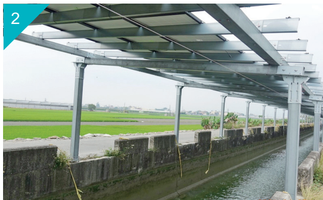
2 彰化二林 (大排, 地面型), 使用熱浸鍍 5% 鋁鎂鋅鋼板 Erlin Township, Changhua County (Ditch, Ground type) Hot-Dip 5% Al-Mg-Zn Coated Steel Sheet
